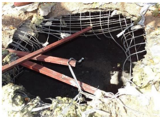
Figure 49.D.4 Entry point EO1
