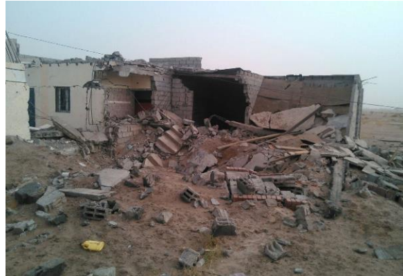
Figure 49.B.3 Armed group suspect's house post-explosion
